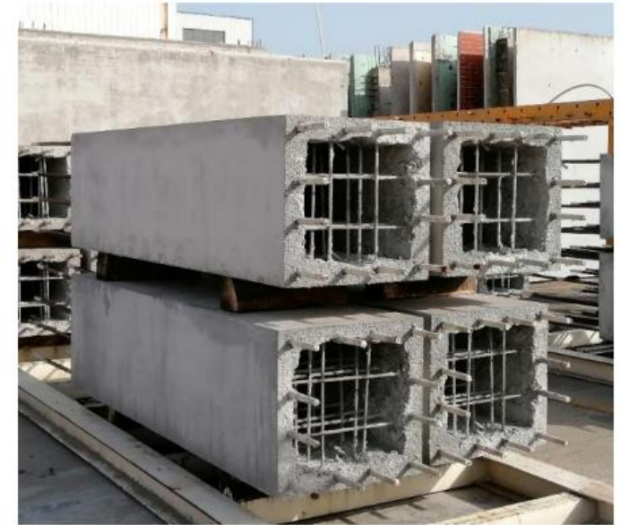
Precast Hollow Core Column
