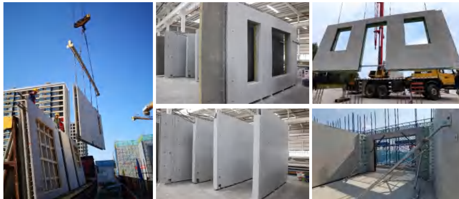
SPCS Cavity External Walls and Internal Partition Walls
